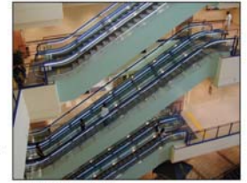
Light Under Handrail
